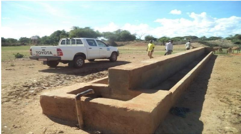
Fig 2: Cattle trough constructed by CISP, Web Kebele Arero
